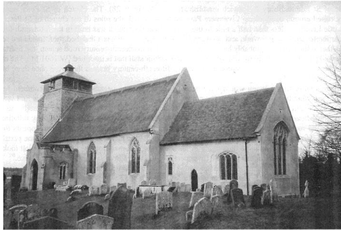
Figure 29. The church of St Peter, Great Livermere, Suffolk in March 2006. The short top to the tower was built after the previous turret fell off in a storm in the 1870s.
