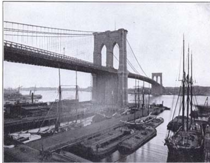
NEW YORK AND BROOKLYN SUSPENSION BRIDGE, NEW YORK CITY
